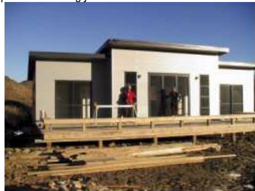
The deck is almost complete on this 3 bedroom bach.
